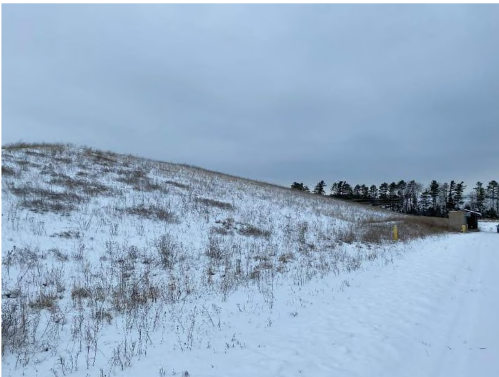
Photo No. 2 – East slope of Landfill No. 3, looking northwest
