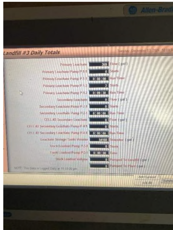
Photo No. 6 – Landfill No. 3 leachate loadout facility screen.
