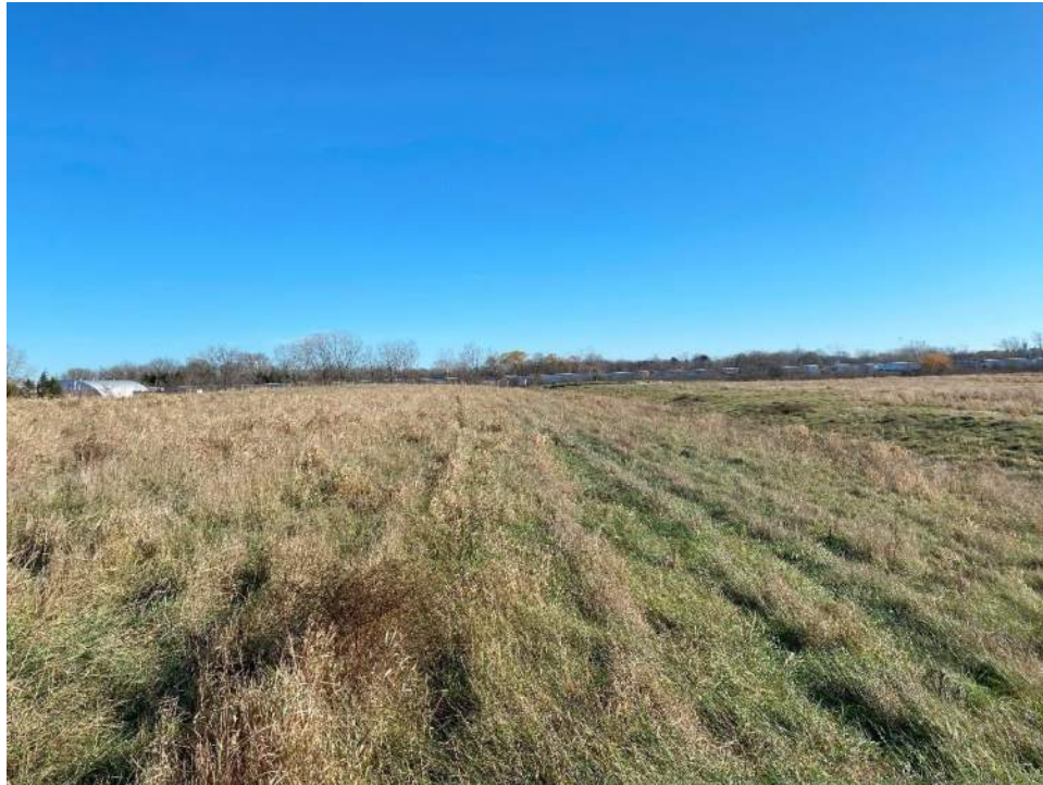
Photo No. 5 – South slope of Cell 1 and perimeter stormwater ditch, looking east.
