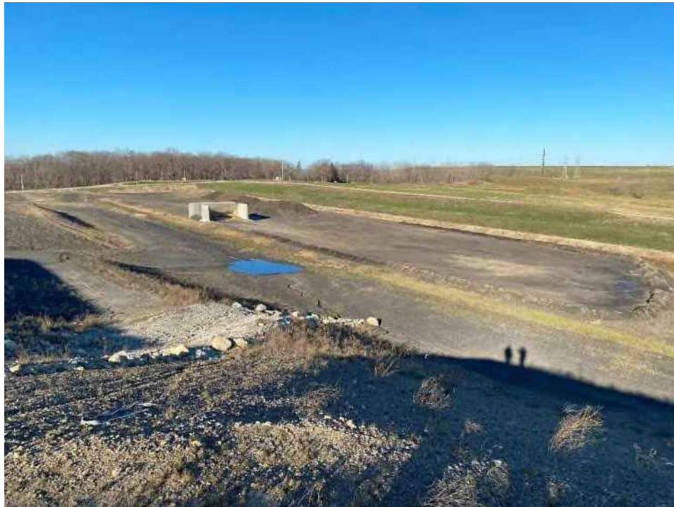
Photo No. 1 – Looking north at active Cells 8 and 10.
