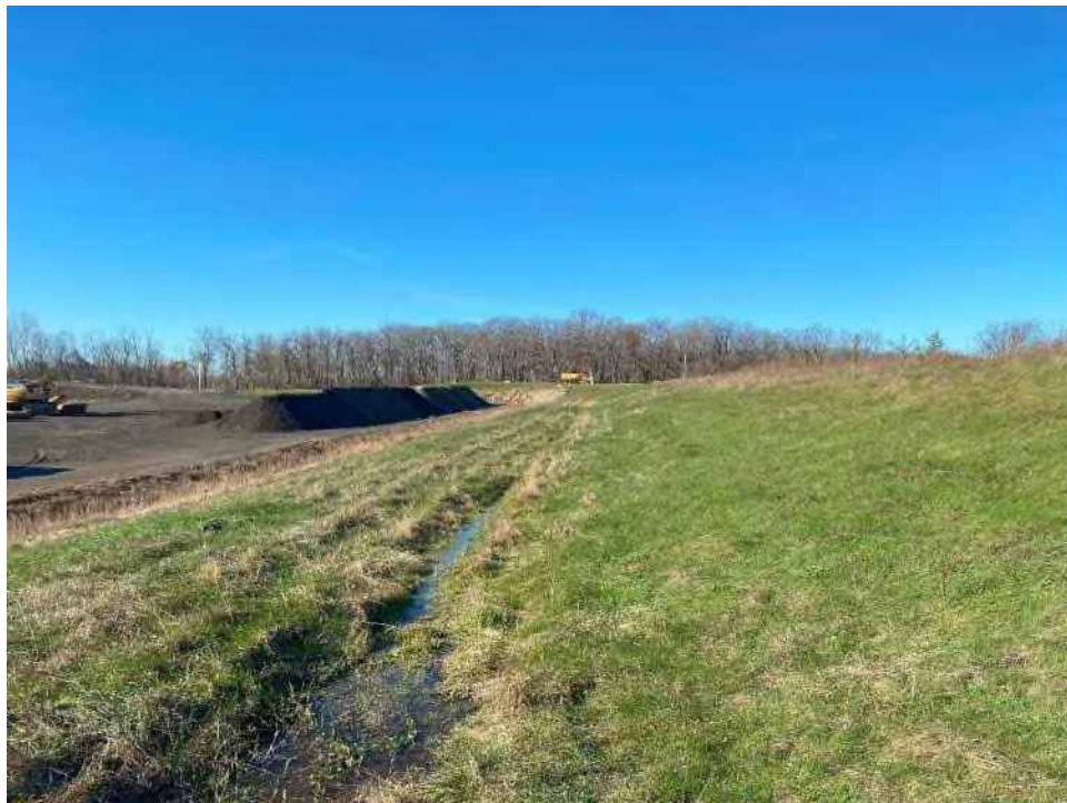
Photo No. 10 – Stormwater ditch north of Cell 10.
