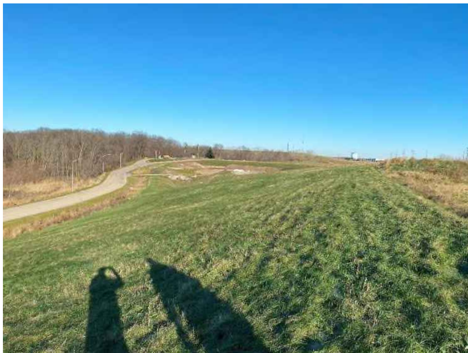
Photo No. 4 – West perimeter berm and stormwater collection ditch, looking north.
