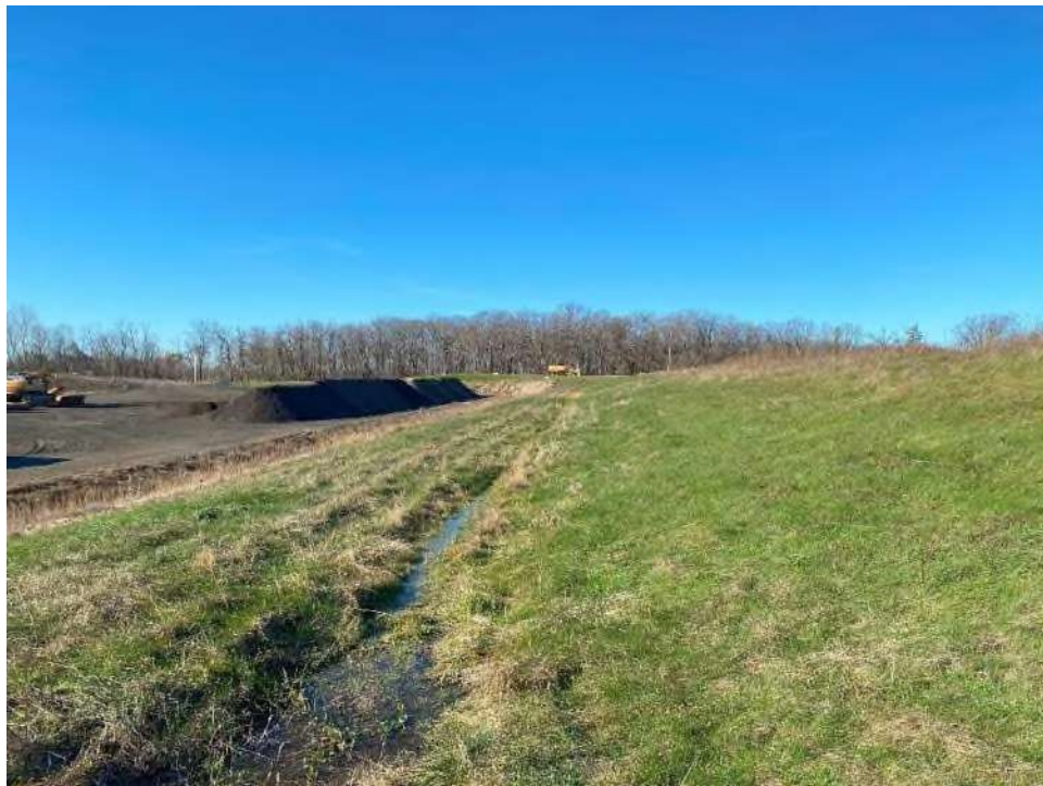
Photo No. 10 – Stormwater ditch north of Cell 10.
