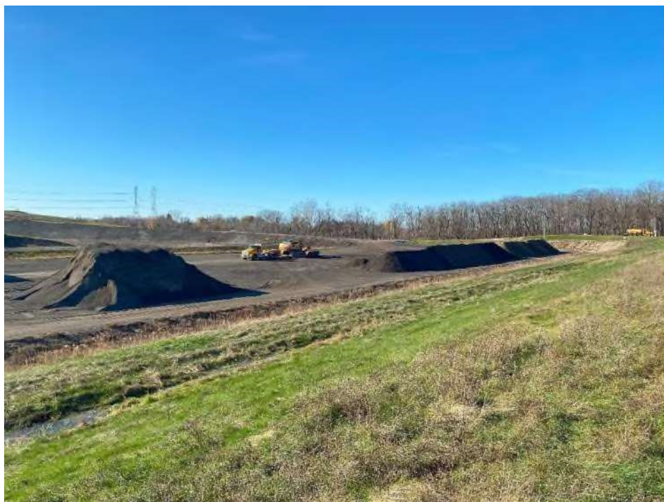
Photo No. 8 – Cell 10 active area. Contractor notified that piles need to be graded and compacted.
