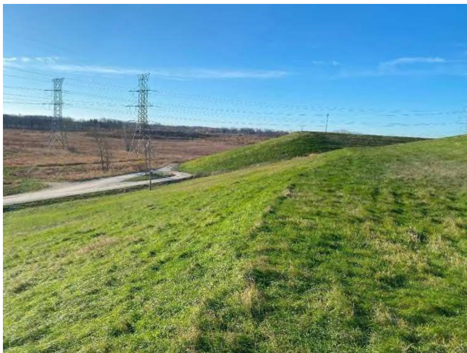
Photo No. 6 – East perimeter berm, looking south.
