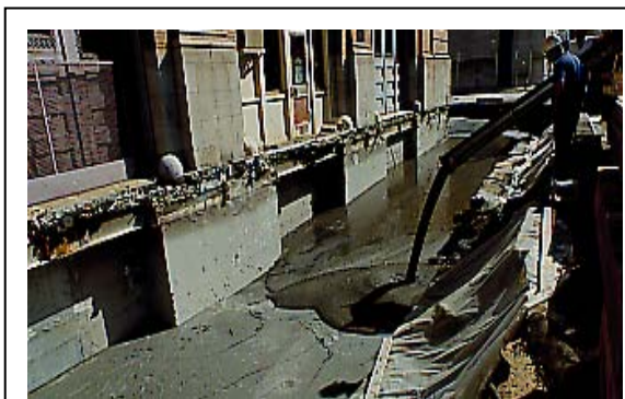
Figure 5-15: CLSM being placed in lifts to manage the load on basement walls.
