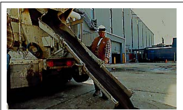
Figure 5-8: CLSM flows into place and completely filled this underground equipment vault.
